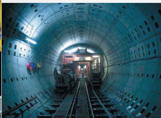
◀ Erector with crossed roller slewing ring for lifting and positioning the lining segments (tubing lining)
