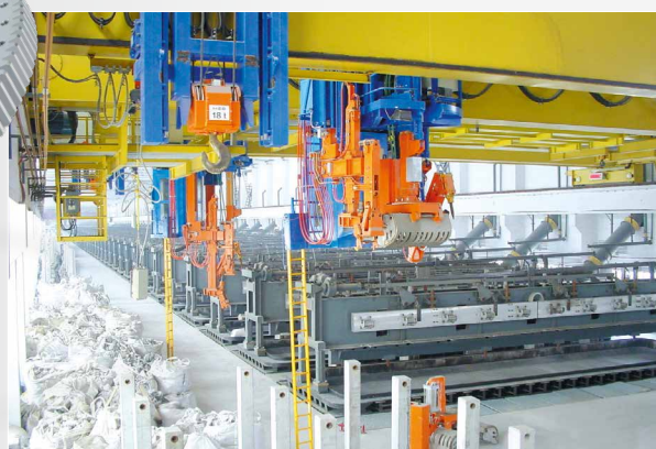
A ball slewing ring with external gear rotates this crane trolley on an aluminum smelter crane
